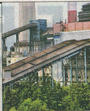
The CESC plant at Budge Budge
